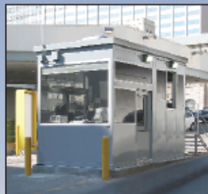
BI-LEVEL TRUCK INSPECTION BOOTH
